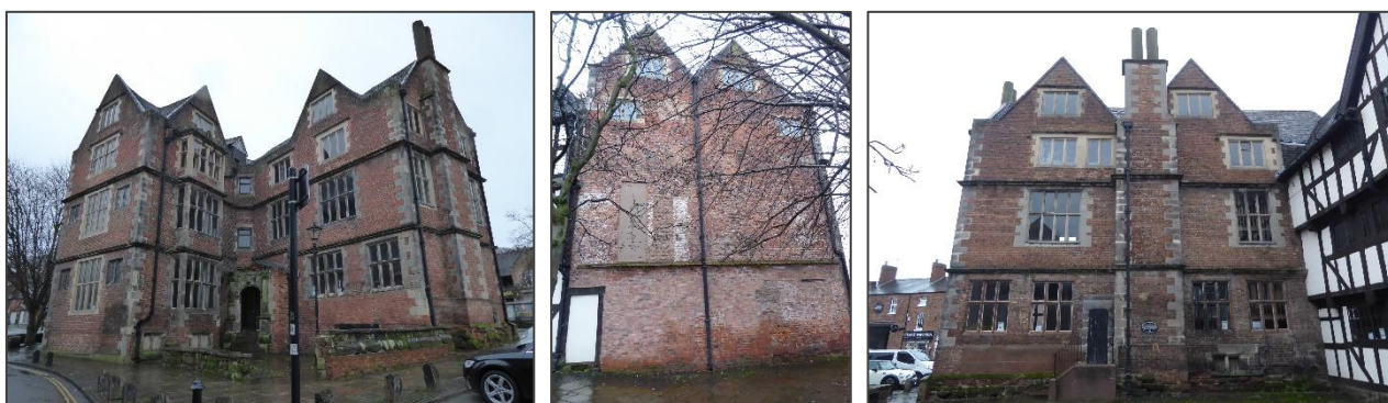
Figure 9: The brick Jacobean style 'Rowley's Mansion' of a north and west wing was added onto the warehouse in c.1616. Left: the principal elevation is formed by the two wings, designed to be seen on the approach from Hills Lane; Centre: the east elevation of the north wing had few features and was built up against another timber framed structure that was demolished in 1930s; Right: west wing, south elevation (Images TDR Heritage 2023).
